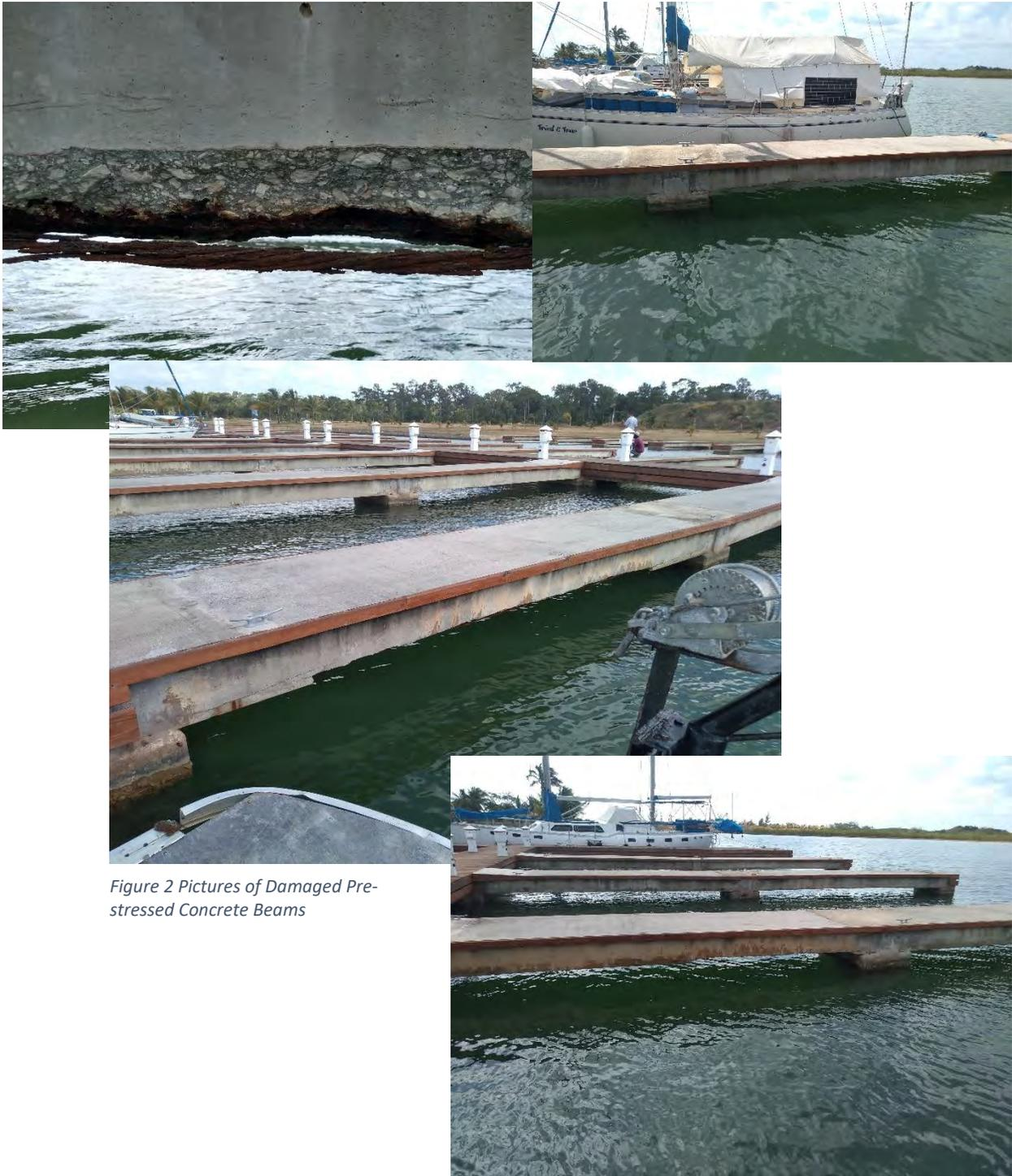
*Figure 2 Pictures of Damaged Pre-stressed Concrete Beams*
